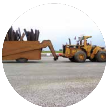
Proof Rolling Test at Kuching International Airport
