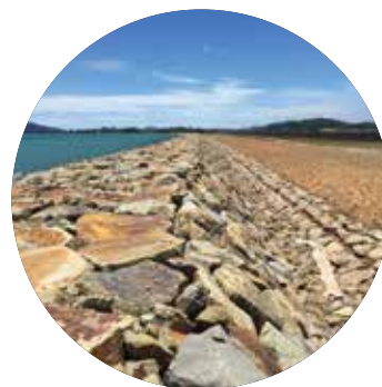
Revetment Works at Kota Kinabalu International Airport
