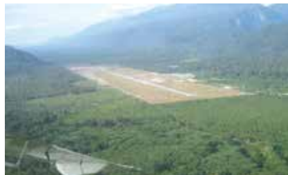
Extension of Mulu Airport, Sarawak
