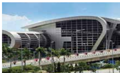
Roof Structure of KKIA Terminal
