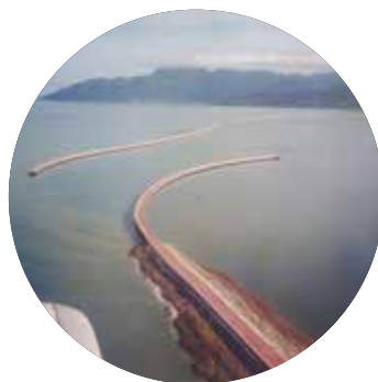
Langkasuka Marina, 8km off-shore breakwater, Langkawi Airport
