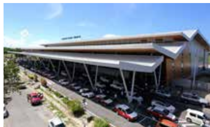
Upgrading of Sandakan Airport Terminal Building
